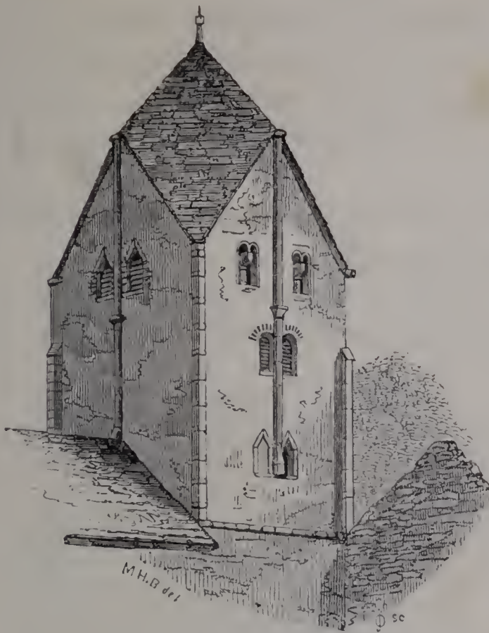
Tower of Sompting Church, Sussex.
